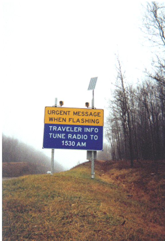
A flashing travel advisory sign such as those being used to manage traffic at the Salt Lake 2002 Olympic Winter Games
